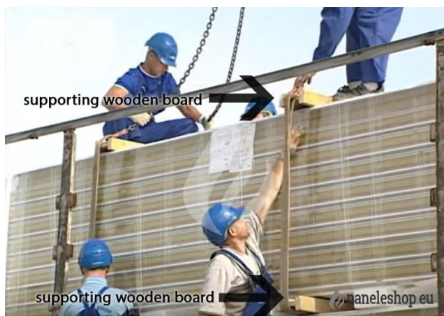
(sample of the supporting wooden board from the bottom and from the top of the package)
